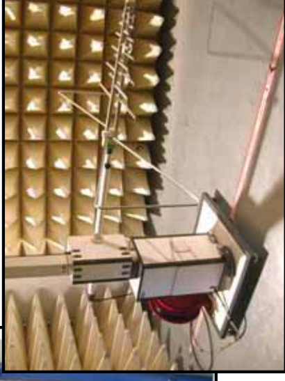
9m * 6m * 6m (EMI Semi-Anechoic Chamber) Testing shall be carried out in accordance with CISPR11
