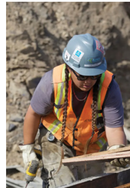
Lori Martin, Mesgi’g Ugju’s’n windpark construction, 2016
