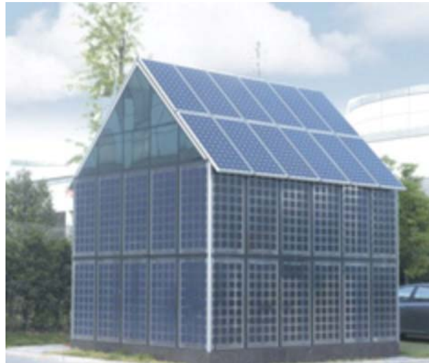
Fig. 46 Glass Conservatory with Double-Glazing Module
