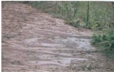
Soil being wash-off
