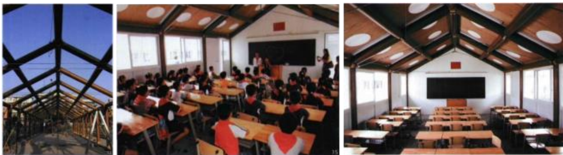
Fig. 1.7 Paper Tube Transitional School Building of Hualin Elementary School, Chengdu
