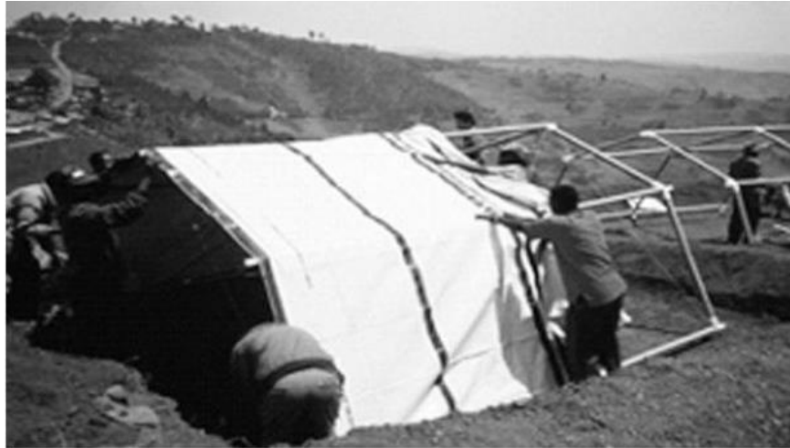
Fig. 1.5 Rwandan refugees set up plastic tents with paper tube support material (Source: Temporary housing after a disaster in an ecological perspective)
