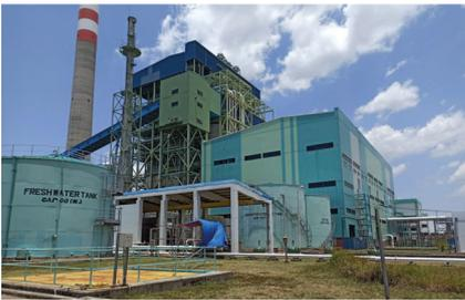
Photo of Coal-fired power plant near Cirebon (West Java), currently the installed capacity is 650 MW and the production of flared CO<sub>2</sub> is about 4 mio. Tonnes per year. In 2022, unit-2 will be on stream with additional capacity of 1,000 MW.
