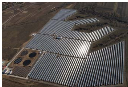
Figure 2-1 Large-scale Ground Power Station
