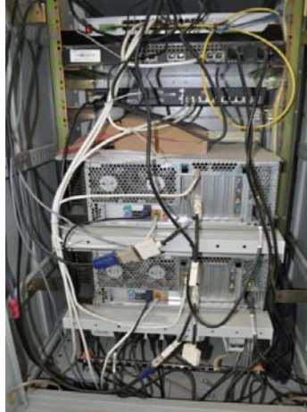
Figure 4-27 Wire Connection Disorder
