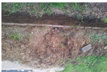
Figure 4-32 Unduly Shallow Cable
