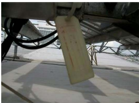
Figure 4-31 Poor ID Durability
