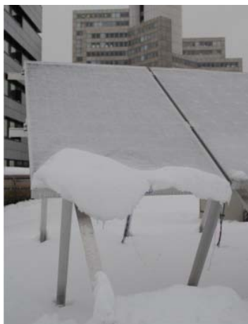
Figure 4-37 Blocking by Snow
