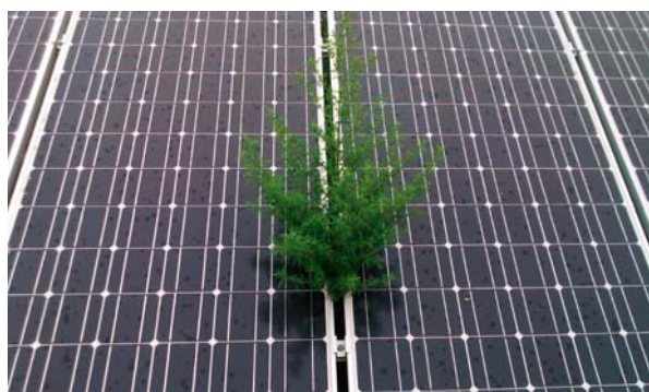
Figure 4-36 Weeds Blocking
