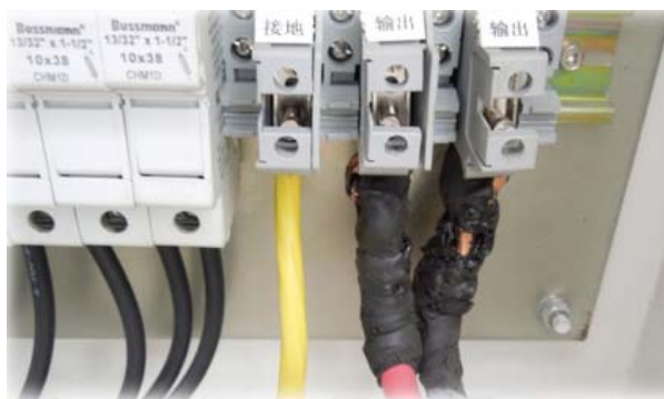
Figure 4-30 Inappropriate Connection
