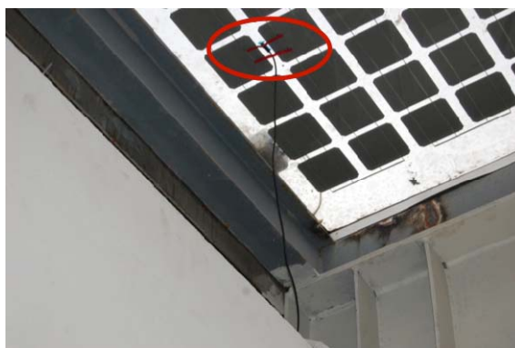
Figure 4-45 Sticking Position Fault of Rear Panel Temperature Sensor
