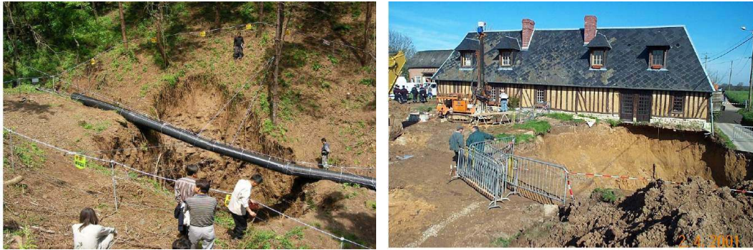
Figure 4.27 Sinkhole crater in Korea (left) and within an urban area in France (ISRM, 2008)
