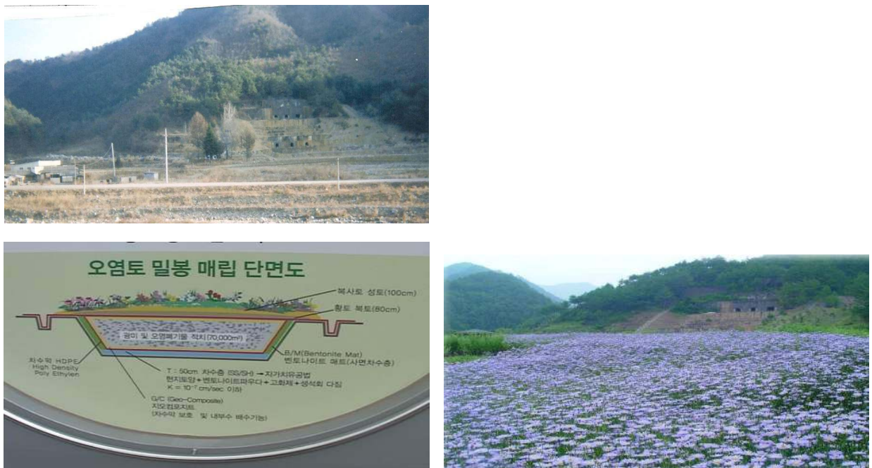
Figure 4.13 Tailing dam of Il-kwang mine that has been reclaimed to form a wild flower park
