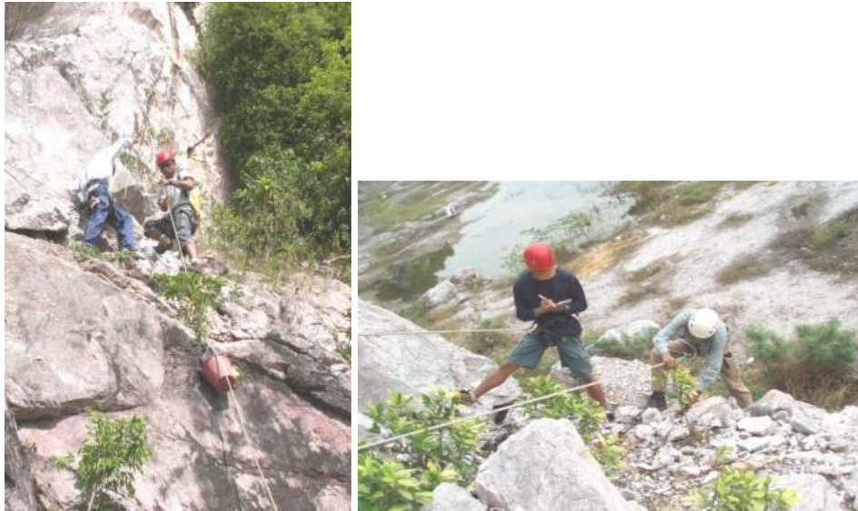
Figure 4.19 Planting of Ficus benjamina at the slope of an abandoned limestone hill quarry (left) and Monitoring of growth, weeding, and fertilization of Ficus microcarpa “Golden” on a bench of an abandoned limestone hill quarry (right).
