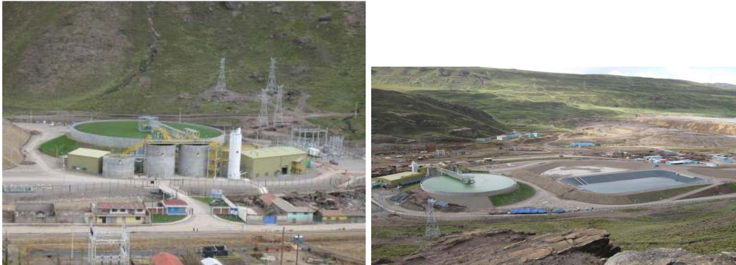
Figure 4.21 High-diversity sludge neutralization system for the treatment of the acidic mine drainage of the Kingsmill Tunnel
