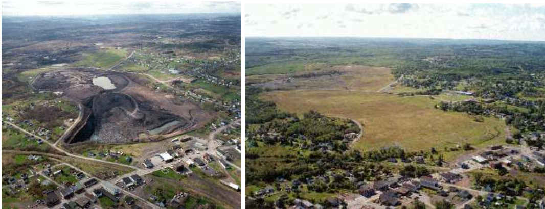
Figure 4.6 Westville surface coal mining site, Nova Scotia before (left) and after (right) reclamation
