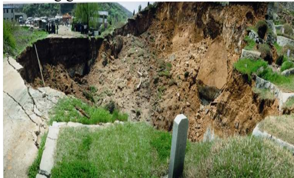
Figure 4.28 Incheon Bupyeong mine in 1993-subsidence and loss of cemetery yard (about 2000 m 2 ) after 6 years of mine closure
