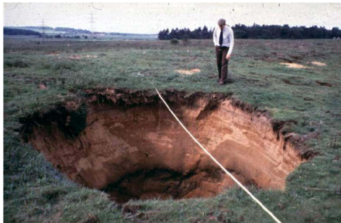
Figure 4.26 Sinkhole crater (ISRM, 2008)
