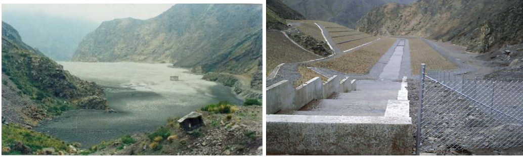
Figure 4.20 Reclamation of tailings deposit of Tablachaca, Peru, before (left) and after (right)
