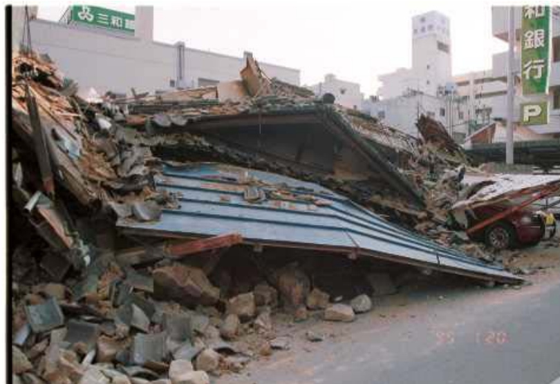
Figure 4.4 Damages of Kobe earthquake (Old wooden buildings)
