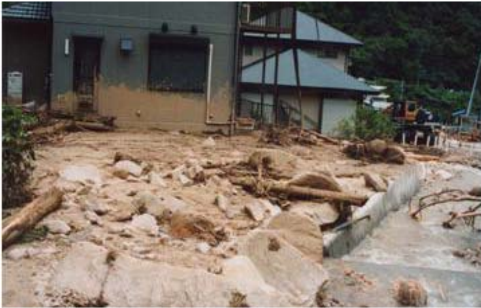
Figure 3.4 Situation of sediment disaster at Hiroshima, 1999(Photo by Ootani)
