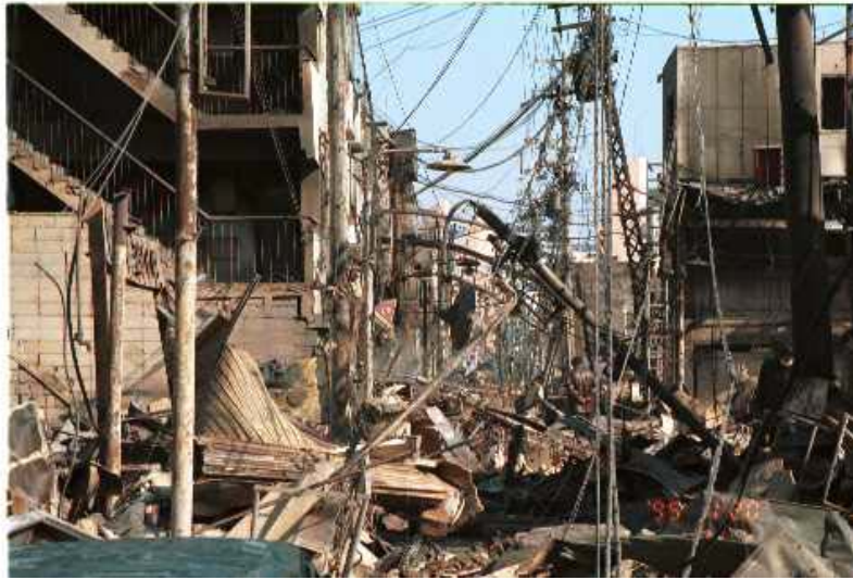
Figure 4.5 Damages of Kobe earthquake (Lifelines)
