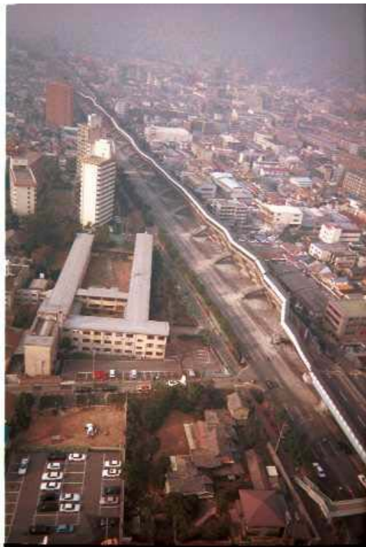
Figure 4.6 Damages of Kobe earthquake (highways)
