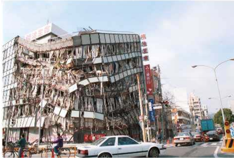
Figure 4.3 Damages of Kobe earthquake (RC buildings)
