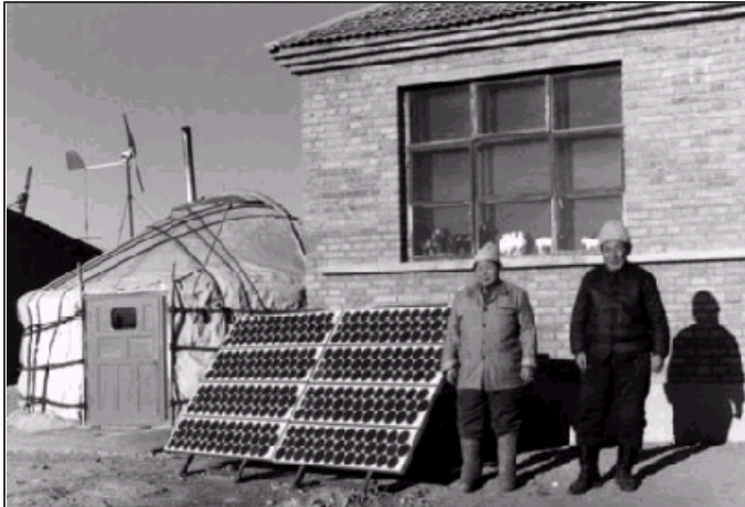
Figure 3: 500-watt PV/wind Hybrid System
