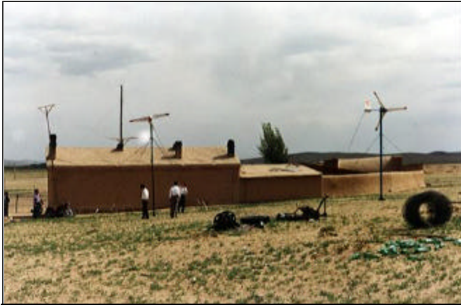
Figure 1: Residential Wind Electric System in China
