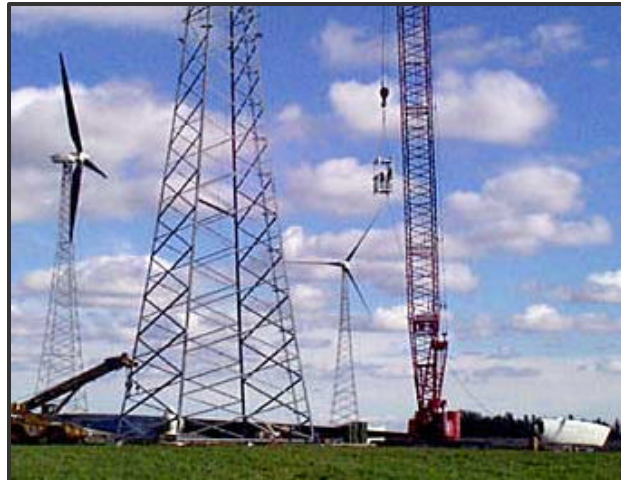
Figure 21. Construction Activities at the Storm Lake Site
