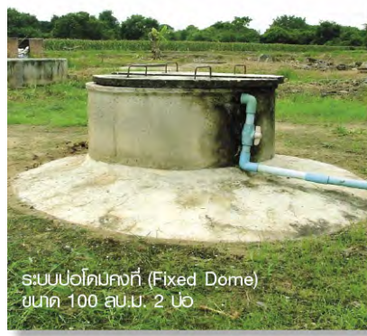
Fig 5. Constructed Fixed Dome at Case Study Site
