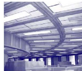
Retrofitting of fluorescent light fittings in the City Administration Centre (CAC).
