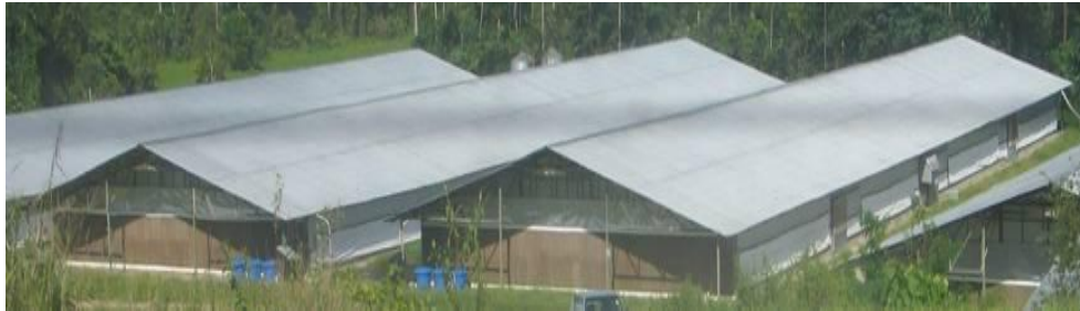
Closed House System for Poultry Farm
