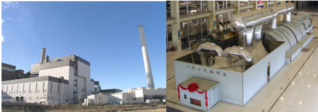
Figure 10.2. Example of firm's product: Steam engine and generator installed in an energy center in the United States
